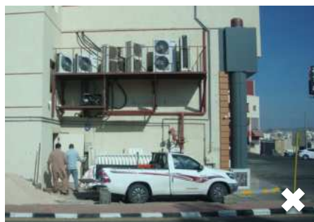
Example of exposed services and utilities
