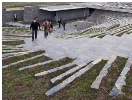
Design respecting the natural terrain Source: Sancaklar Mosque / Emre Arolat Architects, © Thomas Mayer
