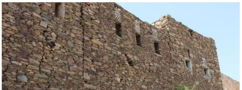
Figure 45 Cluster of buildings forming frontage with small and highlighted openings Location: Al Majared
