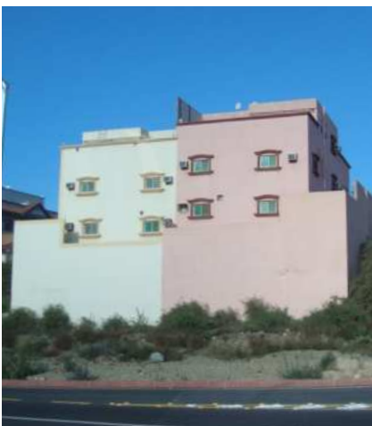
Figure 148 High retaining walls
