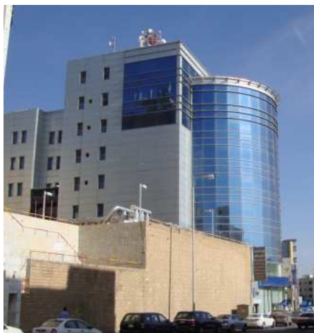
Extensive use of glazing without articulation lacking sense of identity
