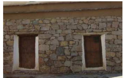
Figure 82 Highlighted door frames and windows Location: Abha
