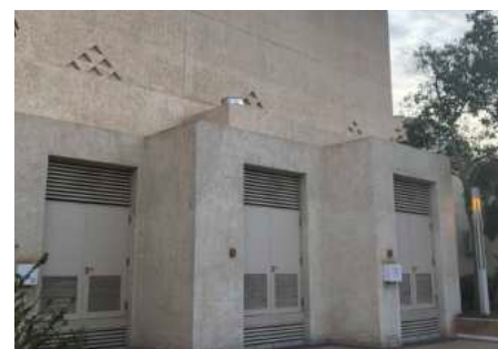
Example of fully screened refusal area integrated within the design of the building
