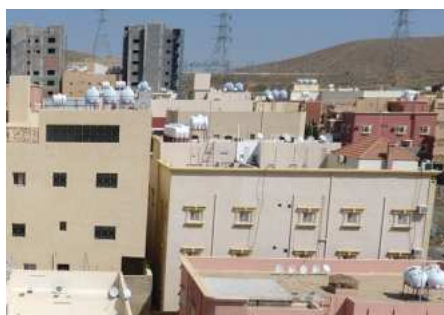
Example of unscreened visible rooftop equipments
