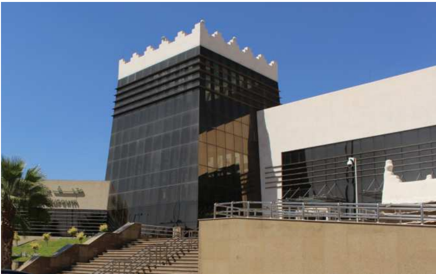
Figure 143 Excessive glazing overwhelming the replica of traditional massing and design
