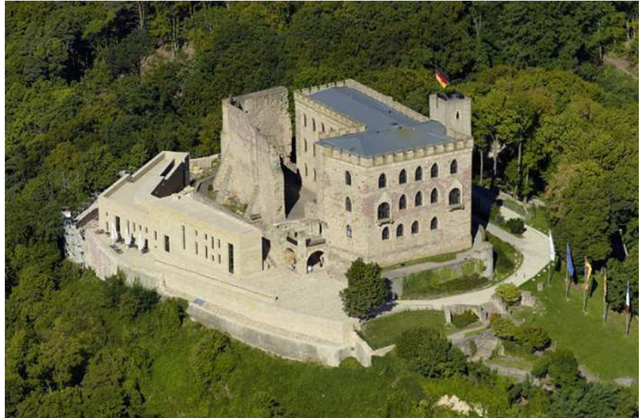
Example of a separate visitor pavilion added to the Hambach Castle in Germany with building materials on the same range color and with similar window rhythm
