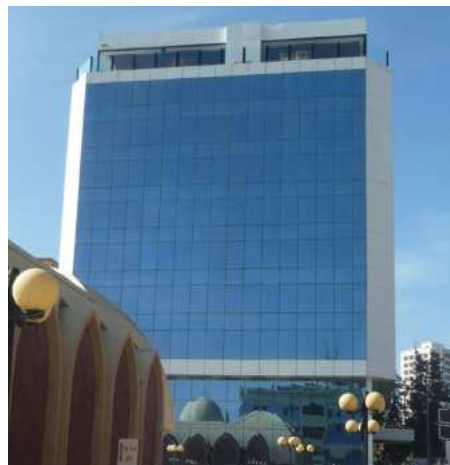
Figure 146 Use of excessive glazing & cladding
