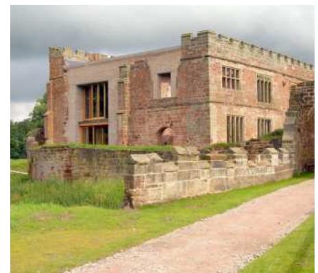
Example of a rooftop reconstruction with harmonious materials for its re-purposing in the UK
