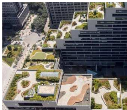
Green stepped terraces with furniture on roof top and appropriately screened equipments
