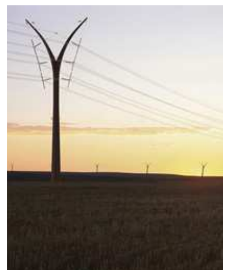
Example of updated design of electricity pylon in Italy
