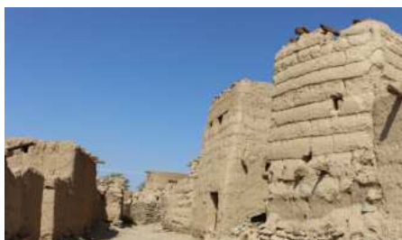
Figure 91 Narrow alleys between buildings Location: Tathleeth
