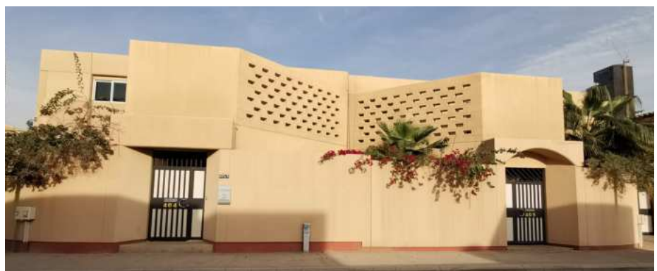
Example of screening elements included into the overall architectural design in terms of material, color and pattern
