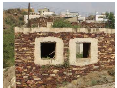
Figure 44 Openings highlighted with white plaster Location: Mahayel
