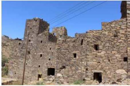
Figure 77 Facade breaks with vertical volumes Location: Abha
