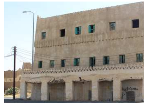
Figure 99 Colonnades and articulated parapets
