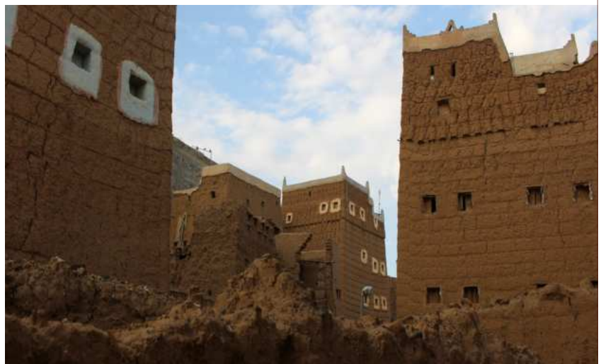
Figure 111 Dhahran Al Janoub old settlements
