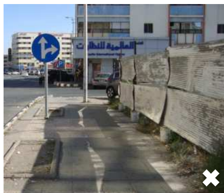
Temporary fencing with corrugated sheets
