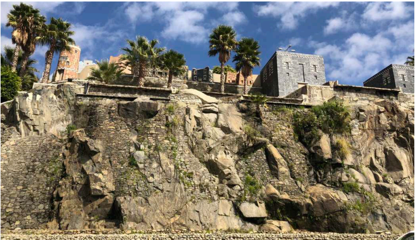
Site photograph illustrating composition of natural rocky feature with constructed retaining in keeping with natural colors and materials and setting of buildings within the slope
