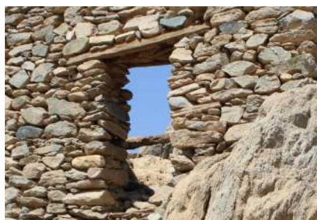
Figure 100 Timber used as tops for the openings
