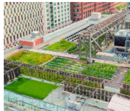
Plantation screening for roof top mechanical elements
