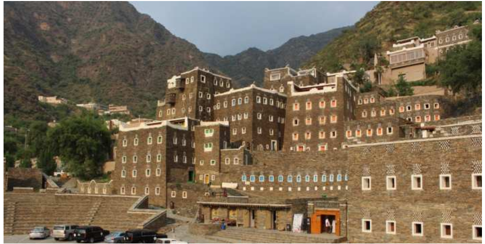
Figure 61 Cluster of buildings forming frontage with colorful openings Location: Rijal Alma
