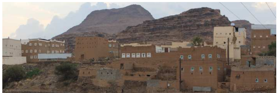
Figure 75 Massing on stepped terraces clustered together Location: Dhahran Al Janoub
