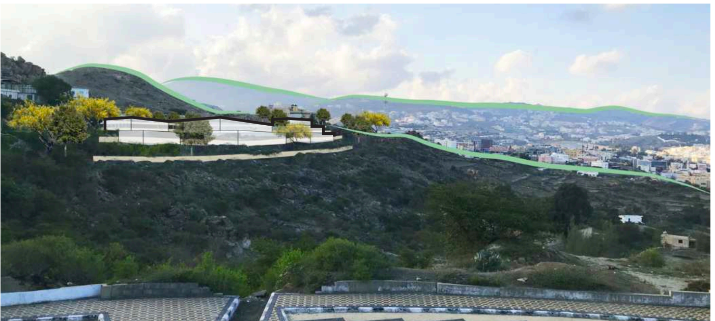
Figure 33 Type 1 visualization from view with modification to reduce impact on the landscape setting, maintaining ridge line, terracing development on slope and sensitive terracing to minimize retaining and erosion, undertaken as part of a 2 Point Study
