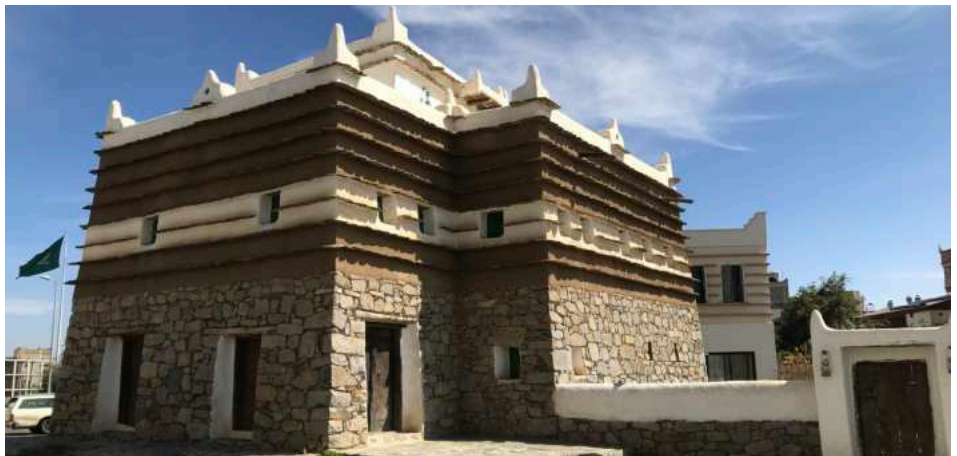
Figure 80 Rows of slates for rain protection, material variation at base, parapets for facade articulation Location: Abha
