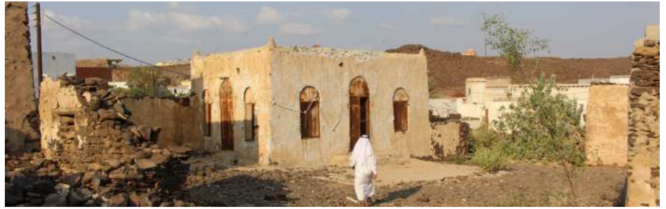
Figure 25 Openings on frontages facing internal courtyard / open spaces
