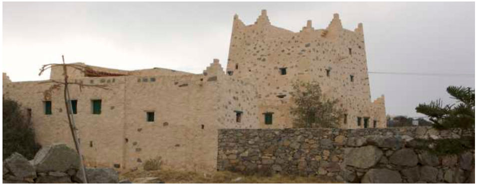
Figure 79 Frontage with limited openings, articulated parapets and integral treatment to all sides Location: Tanaumah
