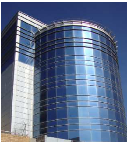
Figure 145 Use of excessive glazing & cladding
