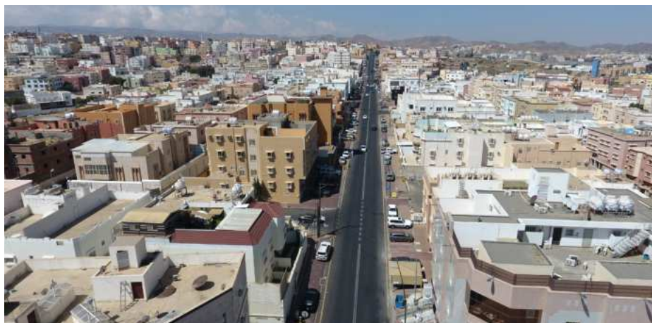
Uniform scale with gradual variation provides street wall and well balanced view
