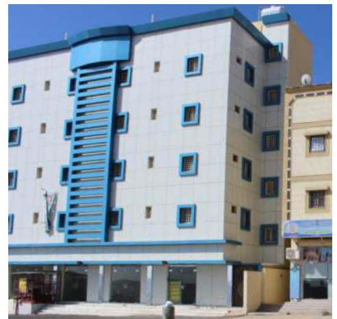
Figure 147 Excessive use of cladding and inapt colors
