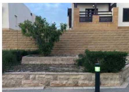
Example of perimeter wall with combination of textures and integrated with landscape
