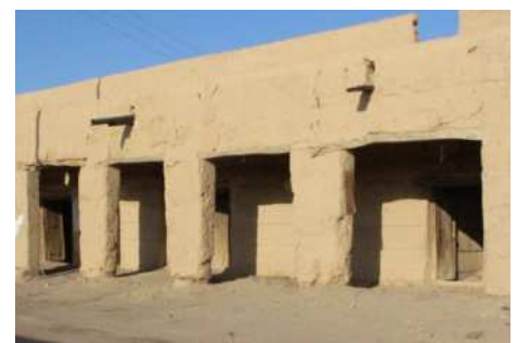
Figure 101 Colonnades on ground floor
