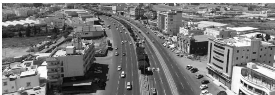
Existing conditions of King Fahd Road in Abha City
