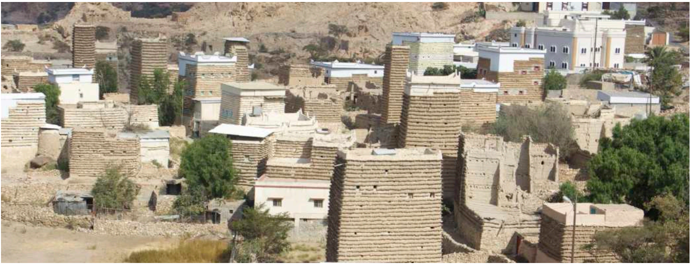
Heritage site, Sarat Abidah
