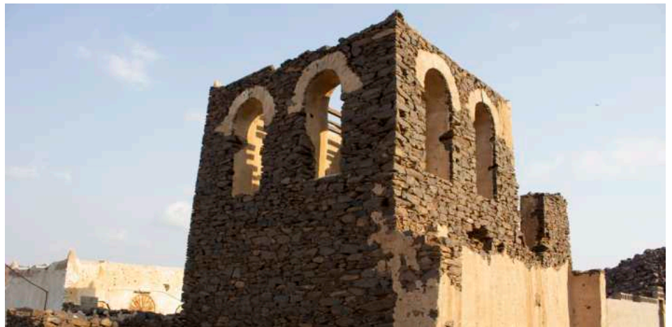
Figure 26 1-2 story with openings on upper floors oriented to bring the sea breeze inside
