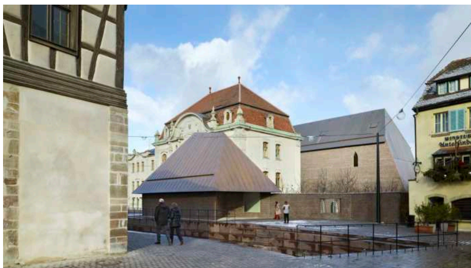
Example of addition reflecting similar features of the historic building in Colmar, France
