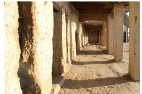
Figure 97 Ground floor colonnades/shading elements
